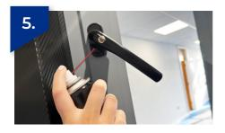
Use a light machine oil on moving handle parts, but not the lock
