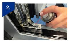
Follow steps 1 to 4 of the window hardware maintenance instructions but remember to lubricate the additional locking and hinge points that are present on a tilt and turn window including along the top and bottom of the window
