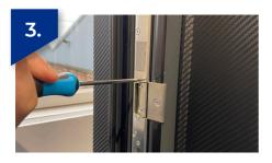
Check the tightness and security of all fixings, tightening as required
